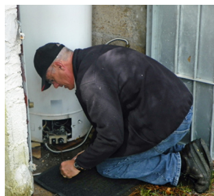
Bottom: Pat DalPorto working on water heaters
