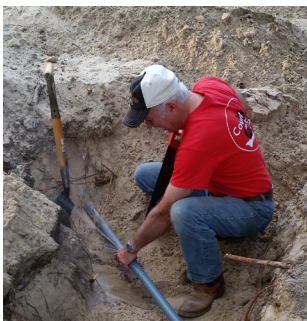
Rick fixing one of many water line breaks
