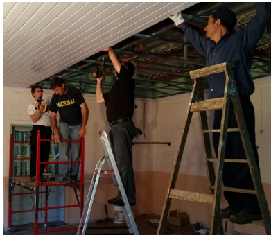
(l-r) Carlos A., Joe, Gaby, & Luis Rios installing the dining room ceiling
