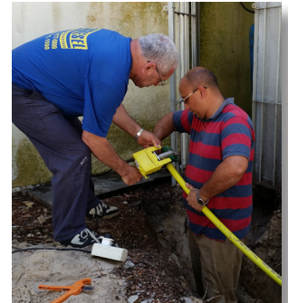
Hector Gomez & the gas man from Hector's church in Rivera splicing gas lines
