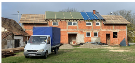
Roof repair on the backside of the new building. The roof will be traditional clay tiles.
