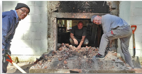
(left) Taking down the original chimney from the side of the dining room.
