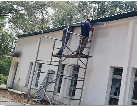
(above) Installing new gutters (for the first time) on the chapel.
