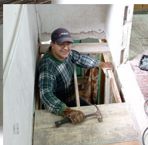
(below) Pedro framing for pouring a floor over the old stairs in the kitchen.
