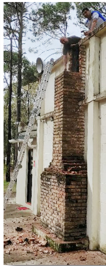
(left) Taking down the original chimney from the side of the dining room.
