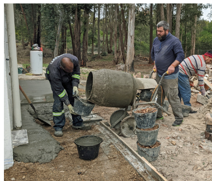
Mixing & pouring the sidewalks
