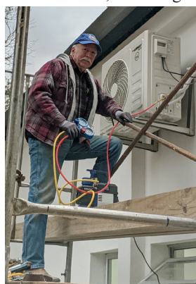
Rick installing an HVAC unit at the chapel
