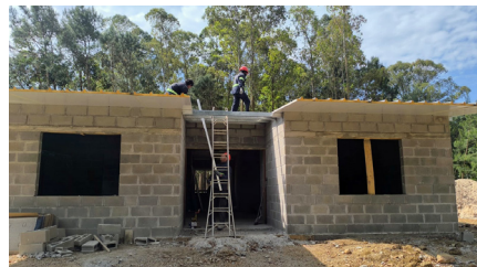
(above) One of the 4 bedrooms (below) Installing the metal roofing
